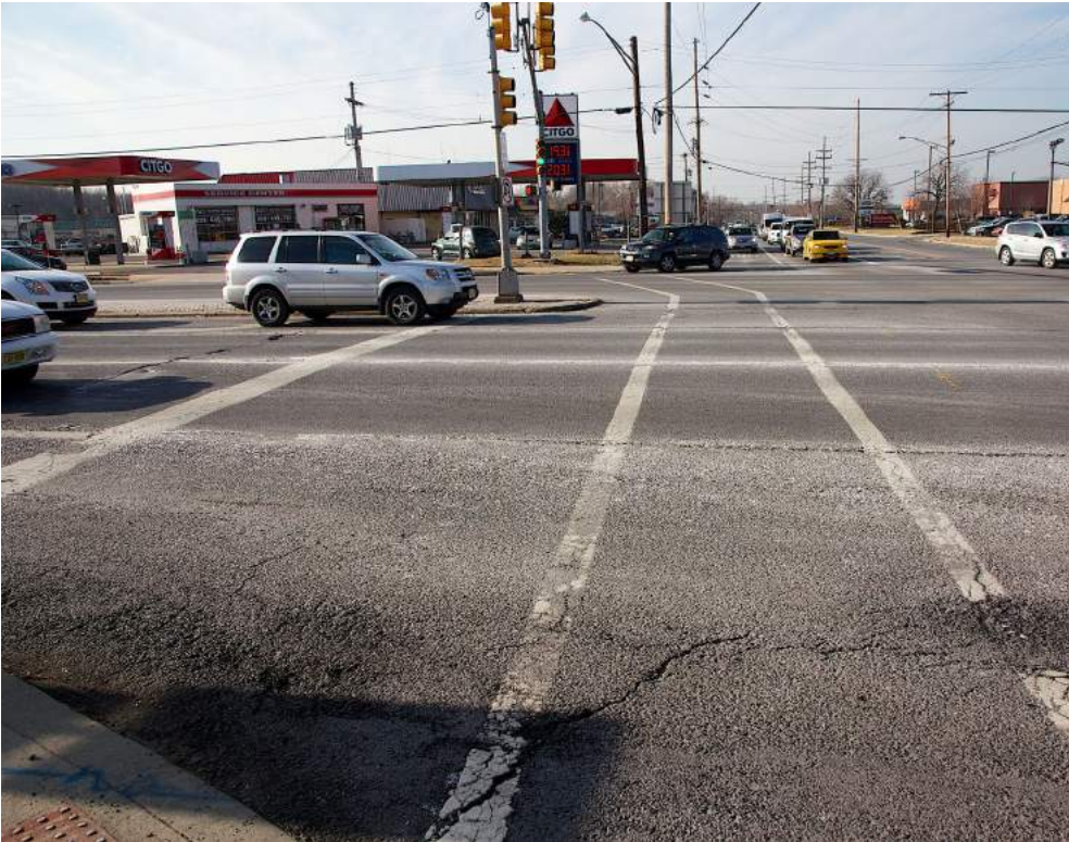
SE corner, facing west
