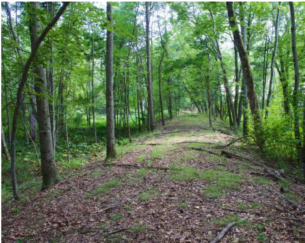
Former rail bed along proposed Union Transportation Trail, near intersection with Airport Road
