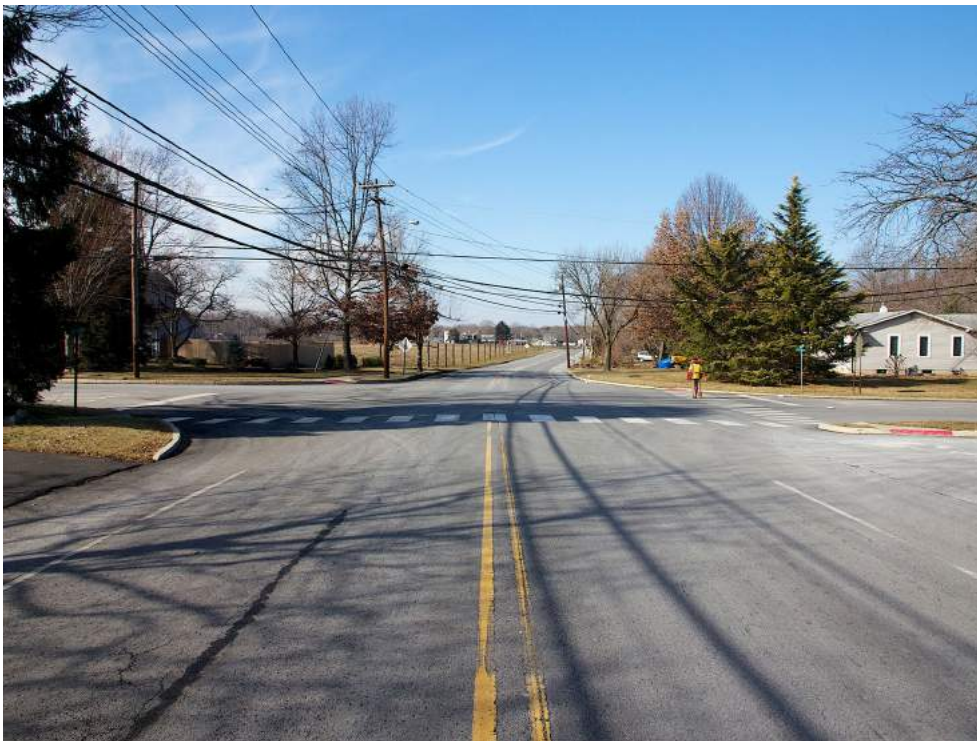
Hickory Corner Road, facing west
