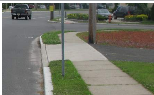
Right: Sidewalk built through driveway
