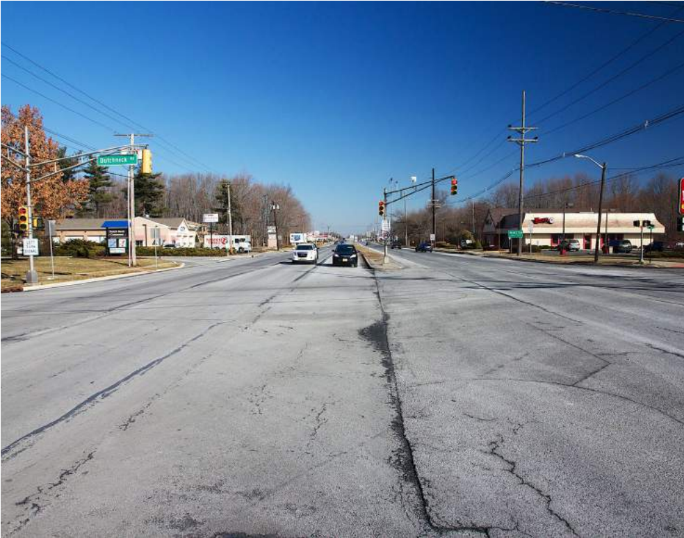
U.S. Route 130, facing north
