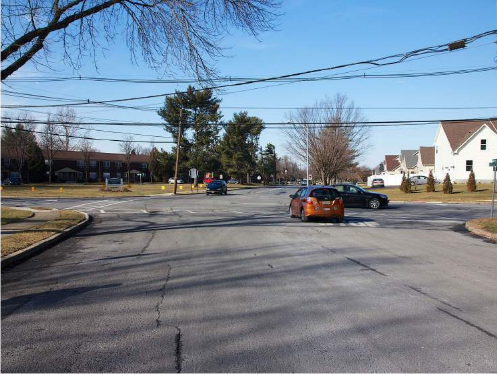
Oak Creek Road, looking northwest
