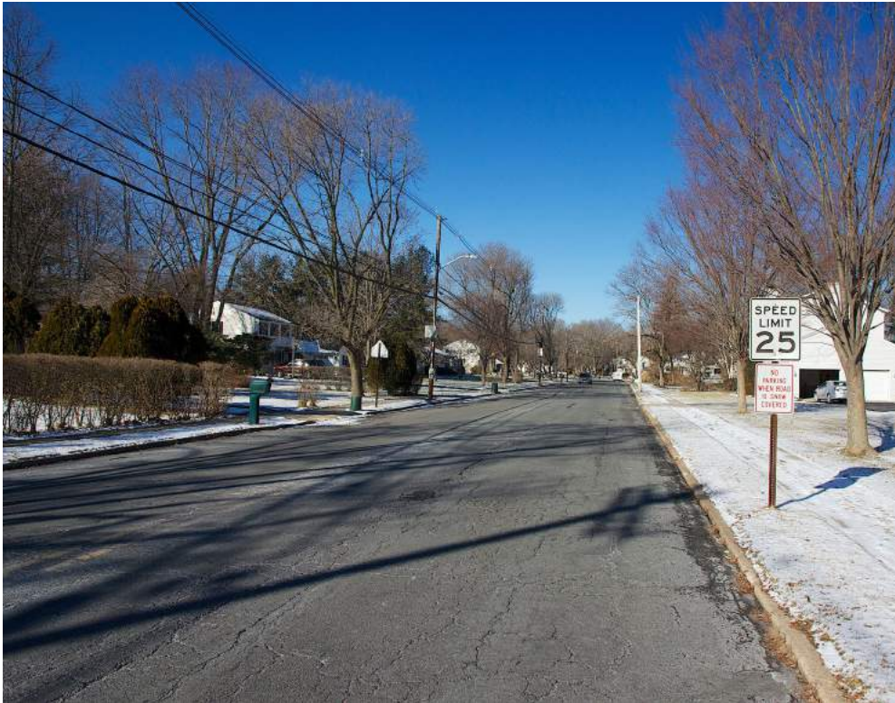
Hickory Corner Road just east of Dutch Neck Road, looking northwest
