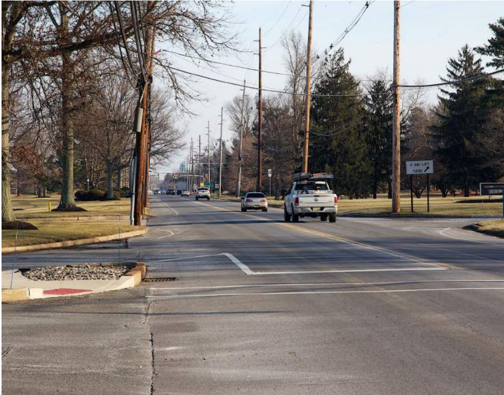
Princeton-Hightstown Road at McGraw Hill, looking southeast
