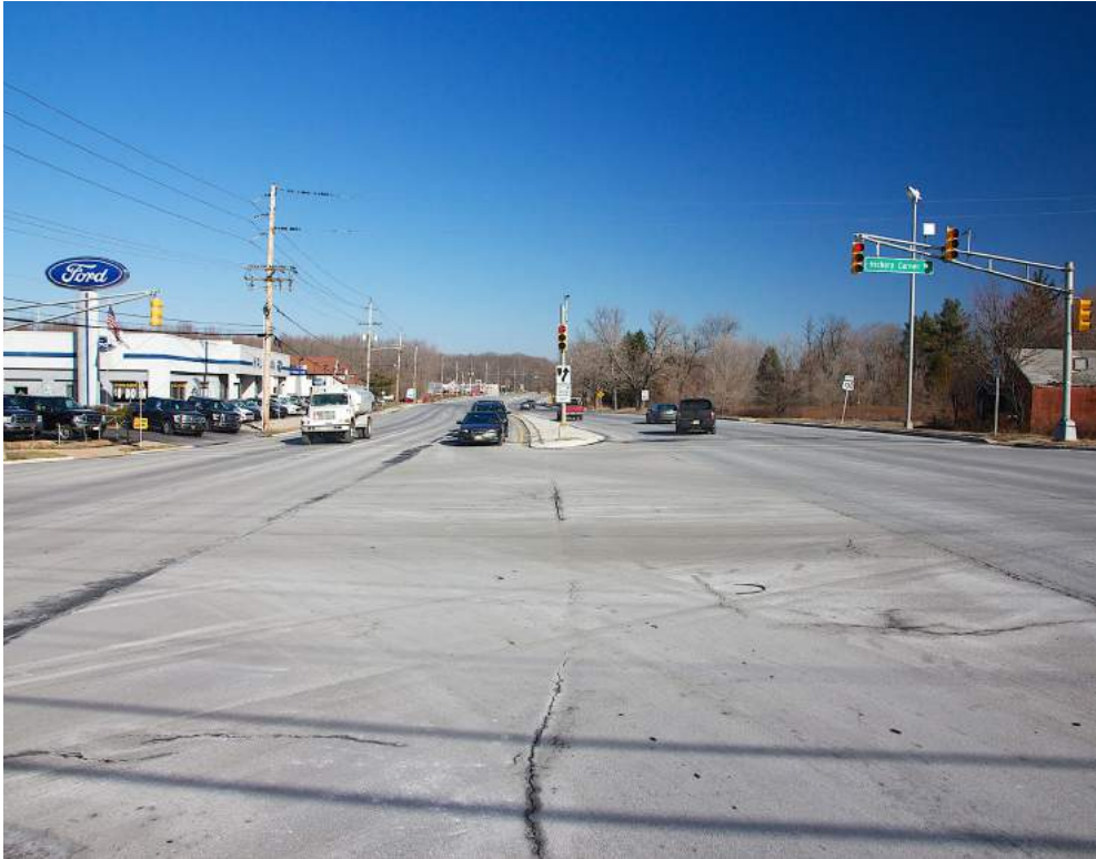
U.S. Route 130, facing north
