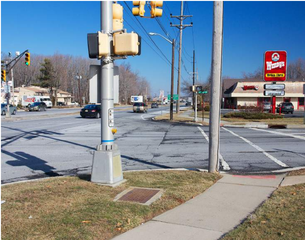
Pedestrian push button not accessible from crosswalk on SE corner, facing north
